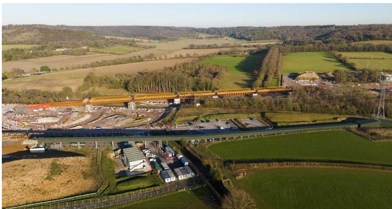
Above: Aerial view of Small Dean viaduct deck in final position across road and railway line in Wendover
