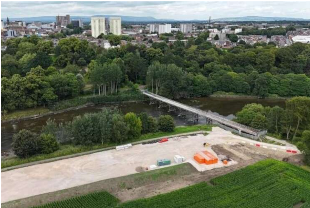
Above: The Old Tram Bridge is coming down
