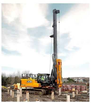
Akela Ground Engineering – part of the Glasgow-based Akela Group – is using a JCB 220X base machine fitted with BSP-TEX JX25-8 piling rig.
