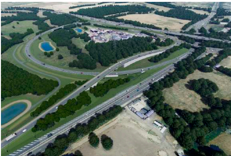
Above: Aerial view of the M25 J28 scheme
