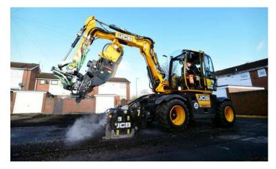
Stoke-on-Trent reports that it has repaired 10,000 m² of road with the JCB PotholePro in just 130 days. Using traditional methods, this task would have taken 1,040 days, it says – nearly three years.
