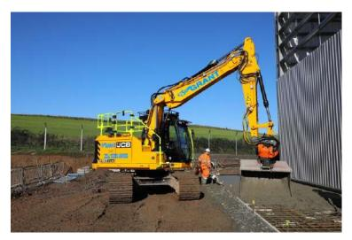
Ayrshire-based Tom Grant Plant's excavator has also been fitted with a Kinshofer Nox TRF14 tilt-rotator for enhanced productivity and versatility.
