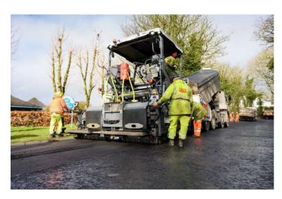
An eco-friendly alternative to bitumen, made from recycled waste plastic, has been approved for use on UK roads.
