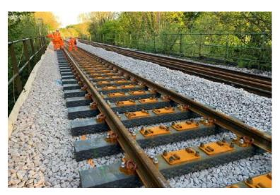
Network Rail has used composite railway sleepers on its main line tracks for the first time.
